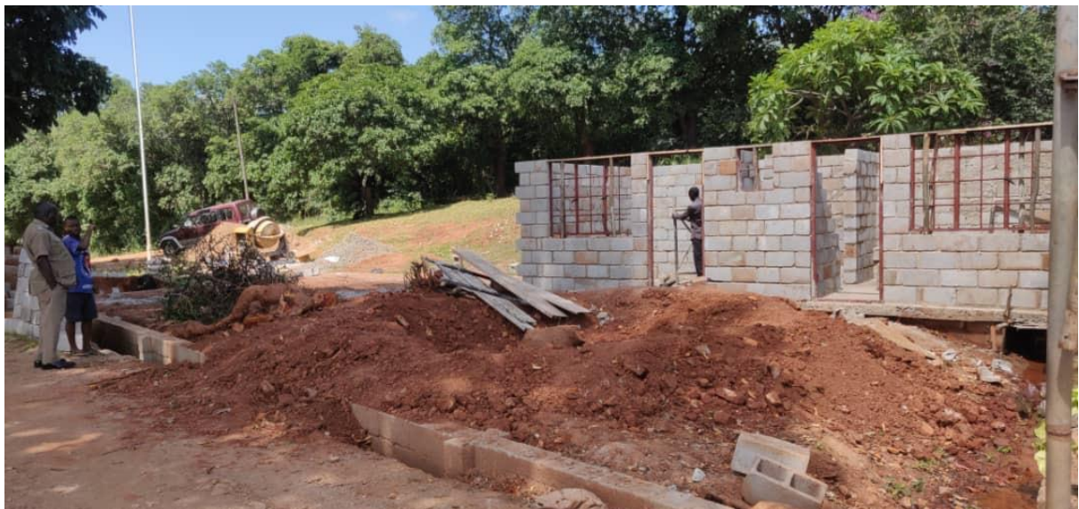
Figure 4 24th March: Another view of the site (Photo WC)
