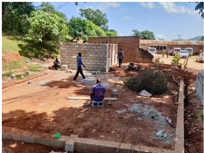
Figure 6 24th March Another View of the Site (Photo WC)
