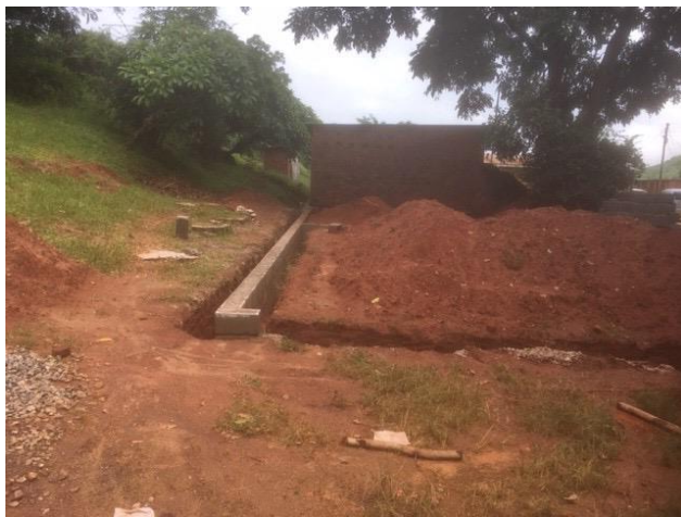
Figure 1 Foundations February 2020 (Photo NM)
