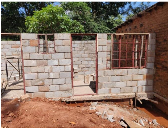
Figure 5 24th March Door and Window Frames in Place (Photo WC)
