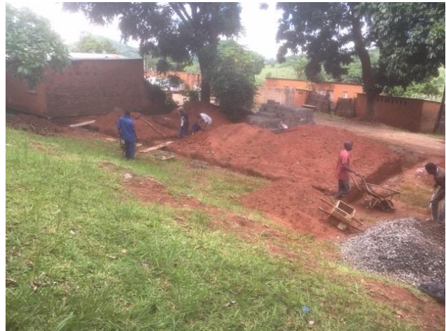
Figure 2 15 th Feb view of Foundations (Photo NM)
