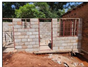
24 th March : 3 pictures of the site including door and window frames in place
