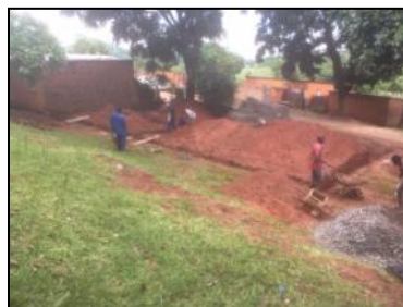
15 th Feb View of Foundations
